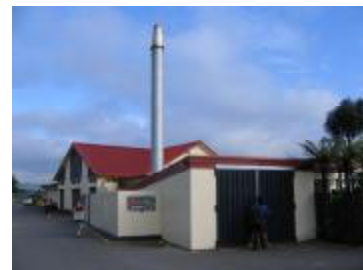
The boiler house and fuel store.
