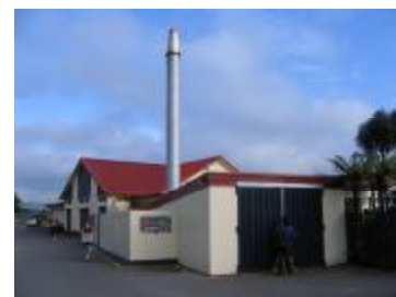
The boiler house and fuel store.
